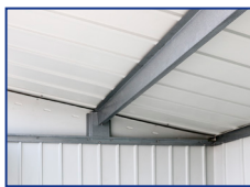
Strong Steel Roof Truss
