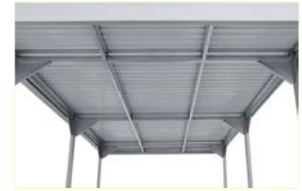
6 Strong metal stanchion & ceiling joist
