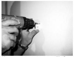
Move unit away from wall and remove Wall Flange from Tube and mount Flange to wall using  $12 \# 10 \times 1-1/4$ " Wall Mount Flange Screws (#3) and Plastic Wall Anchors (#4) if needed.
