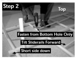
Fastening Horizontal Sliderails (#8) in Rear Grid using 12 - #08 x 3/4" Fastening Screws (#1)
