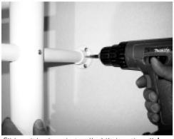
Slide unit back against wall while inserting all 4 Wallmount Extension Tubes (#7) into Wallmount Flanges (#6) and fasten with 4 - #08 x 3/4 Fastening Screws (#1).
