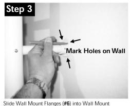
Tubes (#7) Place unit against wall where it is to be mounted and mark Wall Flange holes.
