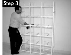
Fasten All Verticals to Horizontals Making sure all joints are pressed firmly together and tight against alignment dimples using 48 - #06 x 1/2" Fastening Screws (#1)
